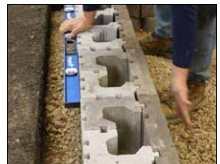
Diagram 4— Assembled units on top of U Start block
