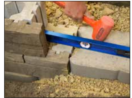
Diagram 7—Stepping up the base
