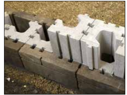
Diagram 21—Second course construction
