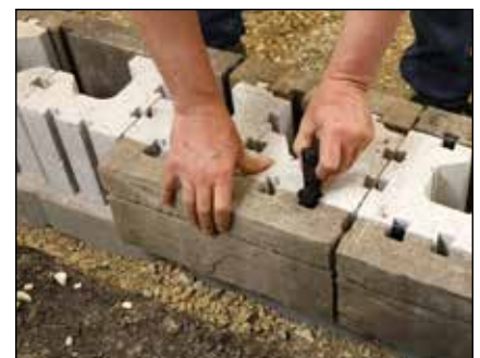
Diagram 20—Placing veneers onto modular block
