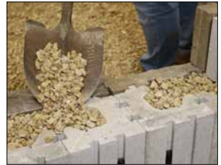
Diagram 5—Fill cores with free draining aggregate
