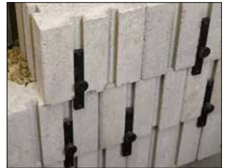
Diagram 6—Lock connector to the block in front
