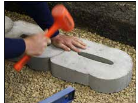
Diagram 3—Lay and level base block
