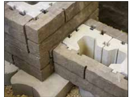
Diagram 23—Ending a wall at a column example
