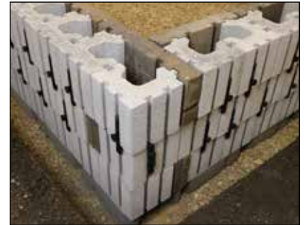
Diagram 12—Corner unit formed
