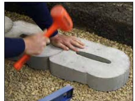
Diagram 19—Lay and level base block
